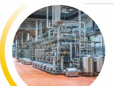
This is Europe's largest dairy powder production plant. We designed and built a factory that can process 3 million litres of milk and whey in 24 hours.
