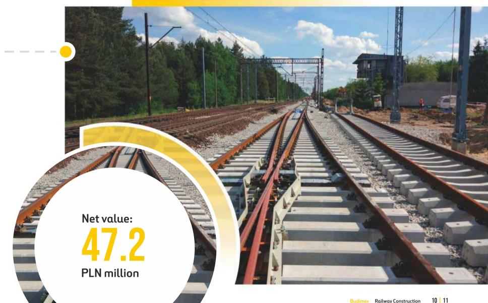
The contract, carried out in a consortium, included the modernization of the Local Control Centre Kutno on the E-20 railway route. The reconstruction included the dismantling of the tracks, reinforcement of the substructure, laying of a new superstructure, and construction of the catenary network and two signal boxes - in Kutno and Barłogi. A new computerized traffic control system was launched at Kłodawa and Barłogi stations.
